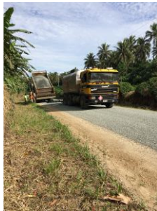
Sealing works underway
